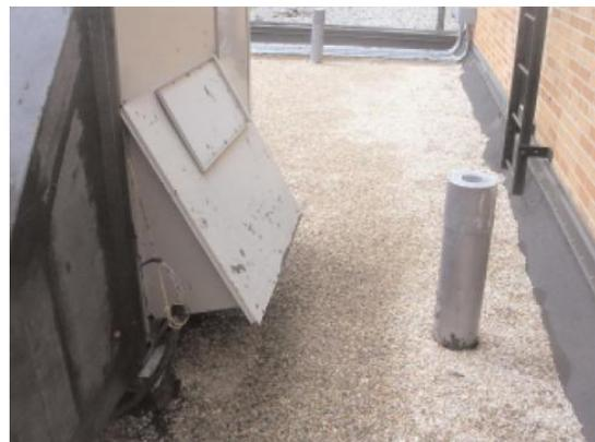
The image on the left shows how exhausted air can be captured by nearby intakes. The image on the right shows a fresh air intake very close to an exhaust.
